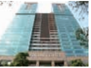
Ho Chi Minh FA Center MITSUBISHI ELECTRIC VIETNAM COMPANY LIMITED
